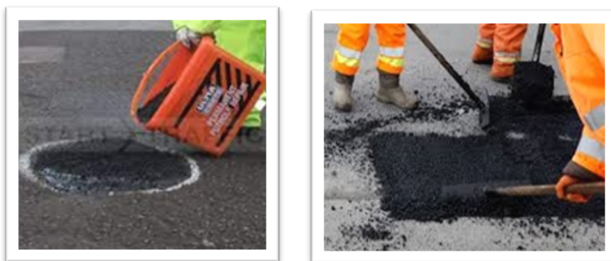
Figure 27. Use of potholes patching materials
