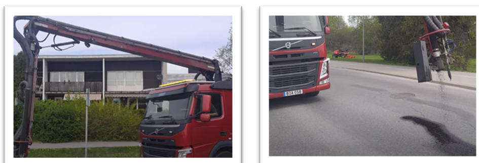
Figure 26. Semi-automatic cracks repairs
