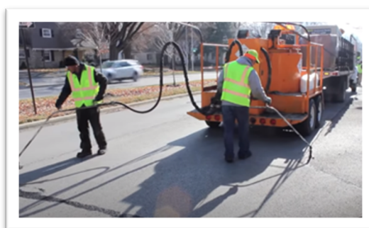
Figure 25. Traditional cracks filling
