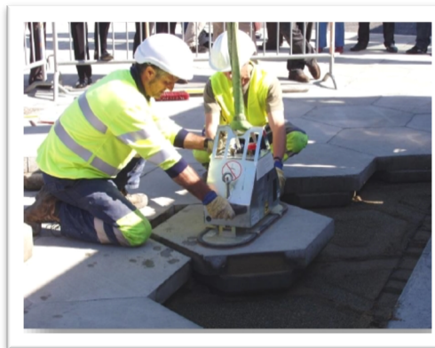
Figure 19. Removal of a RUP slab, using an arm equipped with a suction cup
