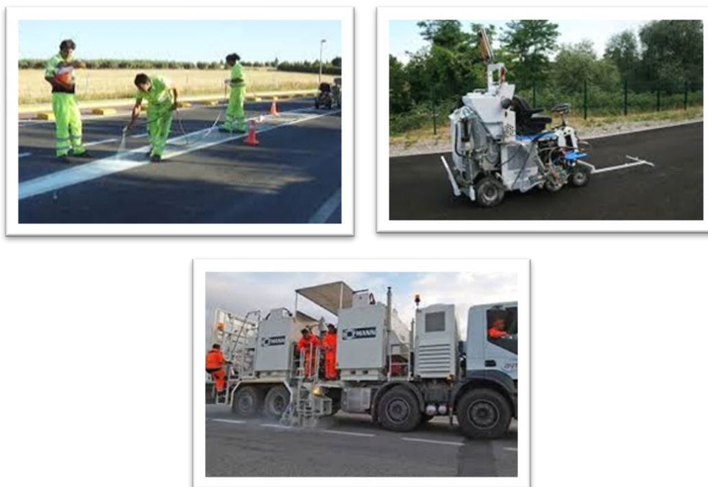
Figure 34. Road marking devices
