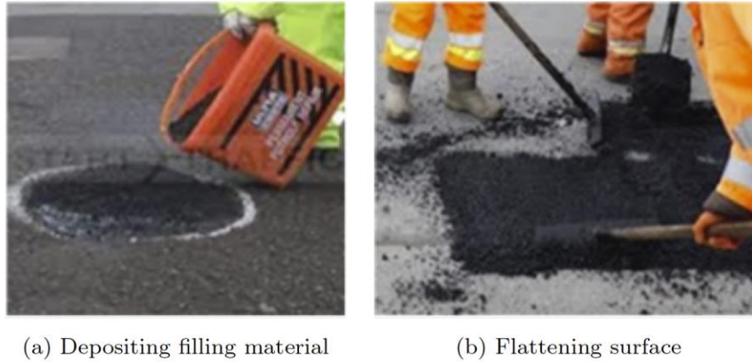
Figure 6: Two steps in the process of fixing a pothole.
