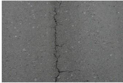
Figure 4: Filling road cracks.
