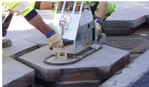
Figure 7: Placing of RUPs.
