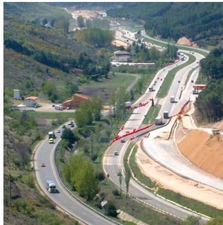
Figure 9: The A-2 motorway
