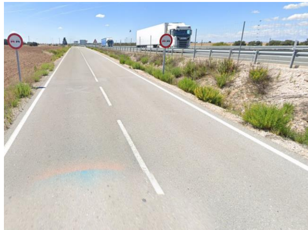
Figure 11: Access Road of La Beltraneja in A-2
