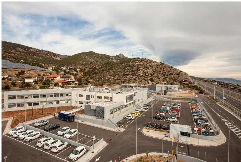
Figure 17: The Olympia Odos Operation and Maintenance Centre (OMC) at Megara
