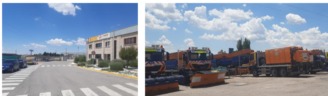
Figure 2: Traffic control centre in Torija
